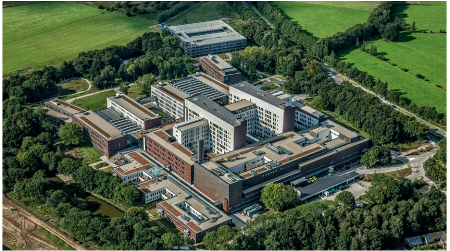
Meander Medical Center (Amersfoort, the Netherlands) is a 600-bed community hospital. Since last year the hospital is concentrated in a beautiful new building, with only single-patient rooms, on the outskirts of Amersfoort. The Radiology Department employs 13 radiologists, 3 nuclear medicine physicians and in total 13 residents. The department operates three 1.5T Philips MRI systems, including Ingenia 1.5T and Achieva 1.5T dStream. ( www.meandermc.nl )
